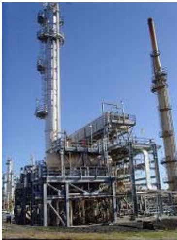
Capture As-Built Data Using 3D Laser Scanning
